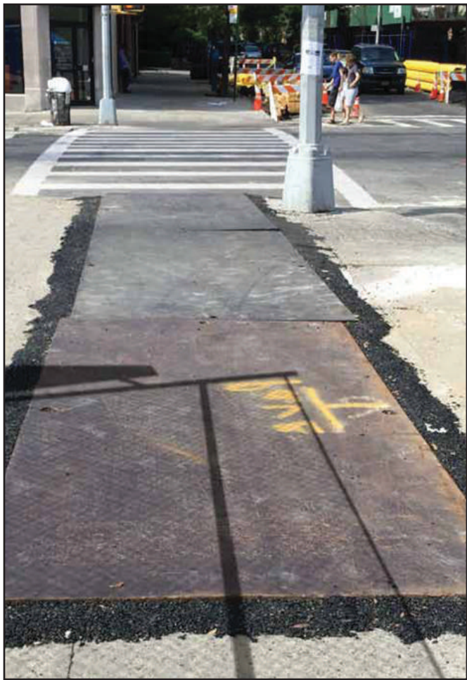
Steel Plates with Cold Patch
