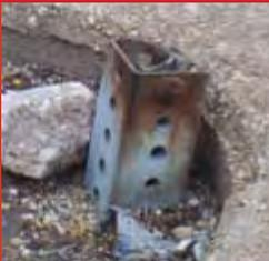
After impact with no breakaway device, the anchor must be replaced. This translates into *more time and expense.*
